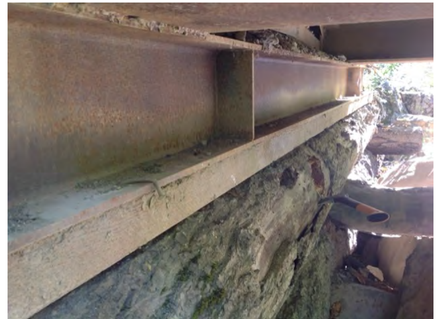
H beam on timber on top of log crib
