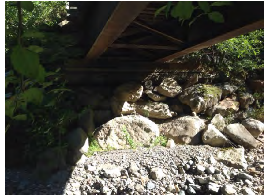
Right Bank Abutment when facing downstream
